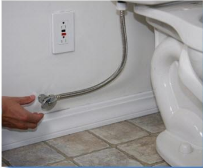
Remove toilet seat & turn off water
