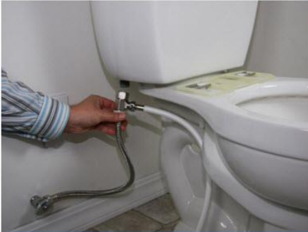
Connect T-Valve & hoses
