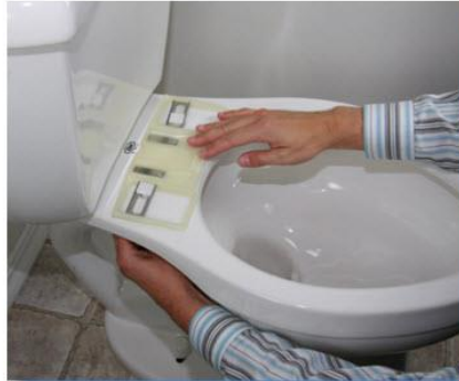
Install mounting plate
